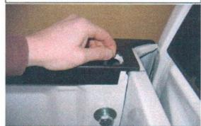
USING 5/8" X 1 BOLT, NUT, LOCKWASHER & FLATWASHER, HAND TIGHTEN BOLT THROUGH THE EXISTING HOLE INTO THE BRACKET.
